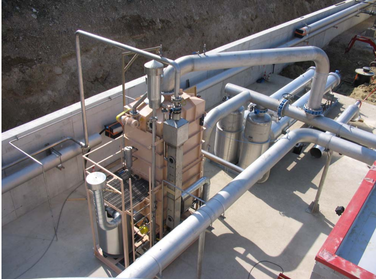
SWOP™ Process at Paris landfill
